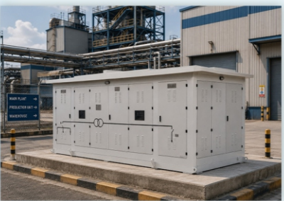
Kiosk and Compact Substation
